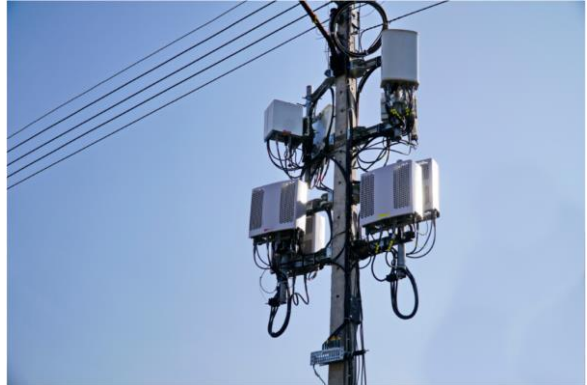
An example of active equipment duplication and the resulting impact on visual pollution. Credit: Shutterstock/kring phromphim
