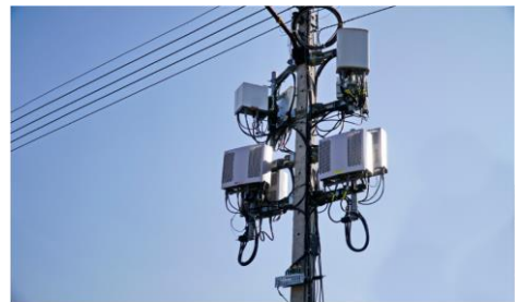
An example of active equipment duplication and the resulting impact on visual pollution. Credit: Shutterstock/kriang phromphim
